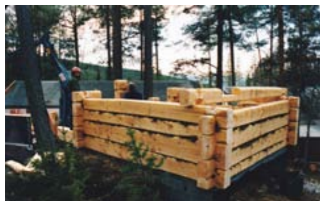
Left: Huge pine logs from old trees with a high resin content were used to make the cogging joints of Paramananda's and moss was laid in between the logs. The whole hut was made entirely with organic materials. Knut Helge Bakos and Johnny Plåt did most of the planning, drawing and construction work, and Knud Larsen designed the interior. Below: A veranda was also built outside the living room of the old building, facing south. Bjørn's father, Ole (right), and younger brother, Trond (left), were carpenters with assistance from Bjørn. All photos: BP.
